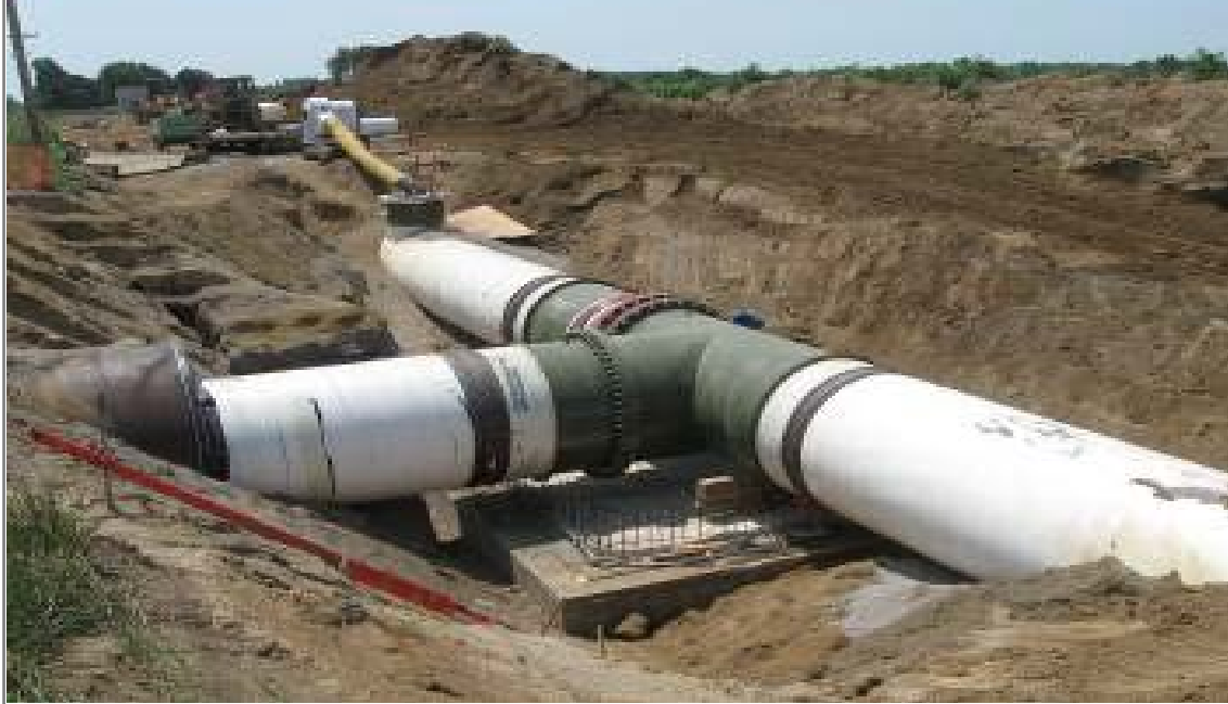
Construction of the raw water line with 72-inch steel pipe
