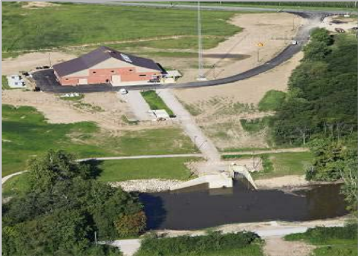
Raw water pump station located by the Scioto River
