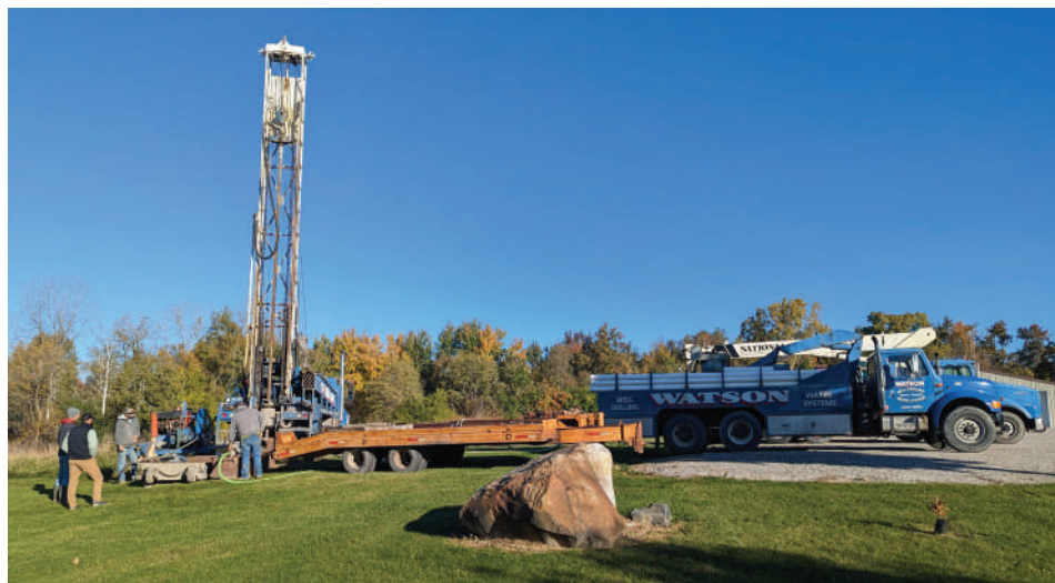
ODNR installed new groundwater-level observation wells at 12 sites as part of this project.
